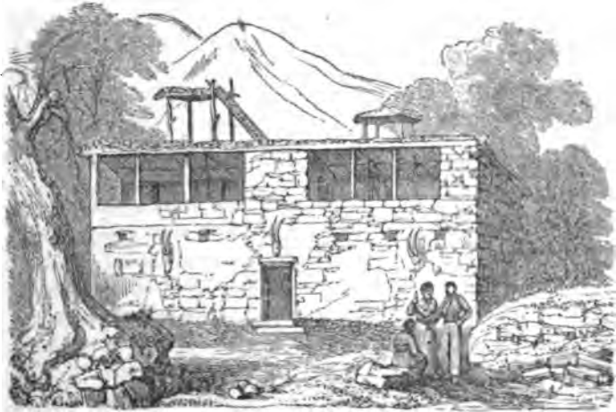
A Nestorian House in the District of Tiyari.
